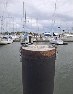
Lengths of timber are to be secured to the top of each pile by fastening the chain with either a D shackle, snap shackle or small length of rope.
